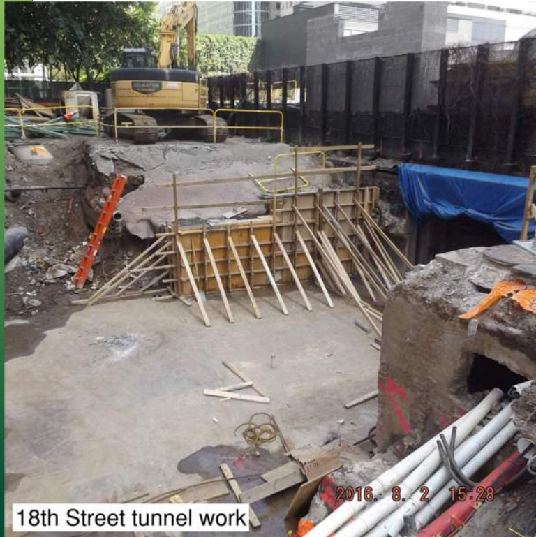
Continued Demolition and Clean up for Proposed Tunnel
