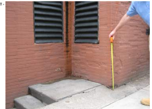
Sterling Building – Cuthbert Street Access
