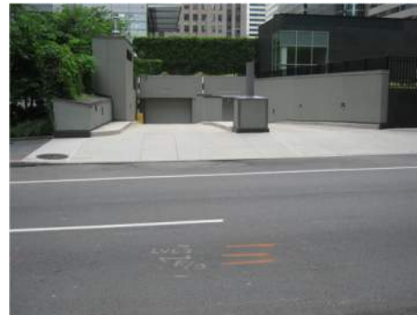
Existing Comcast One underground parking garage ramp
