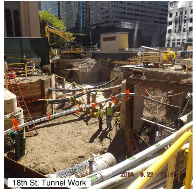
Continued Utility Relocation Work
