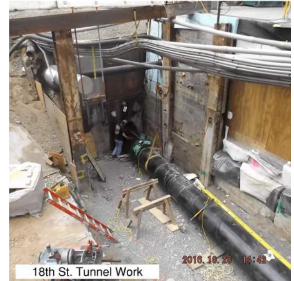
Relocated Steam Line connection into Existing Steam Tunnel
